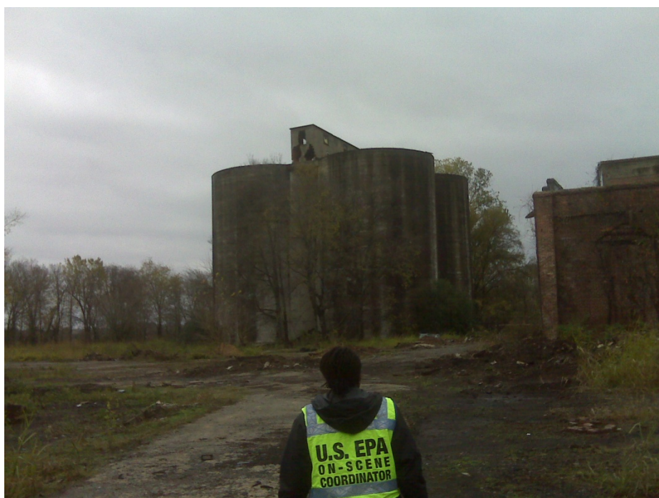
View of four on-site storage silos behind the warehouse at the Former W.R. Grace Facility.
