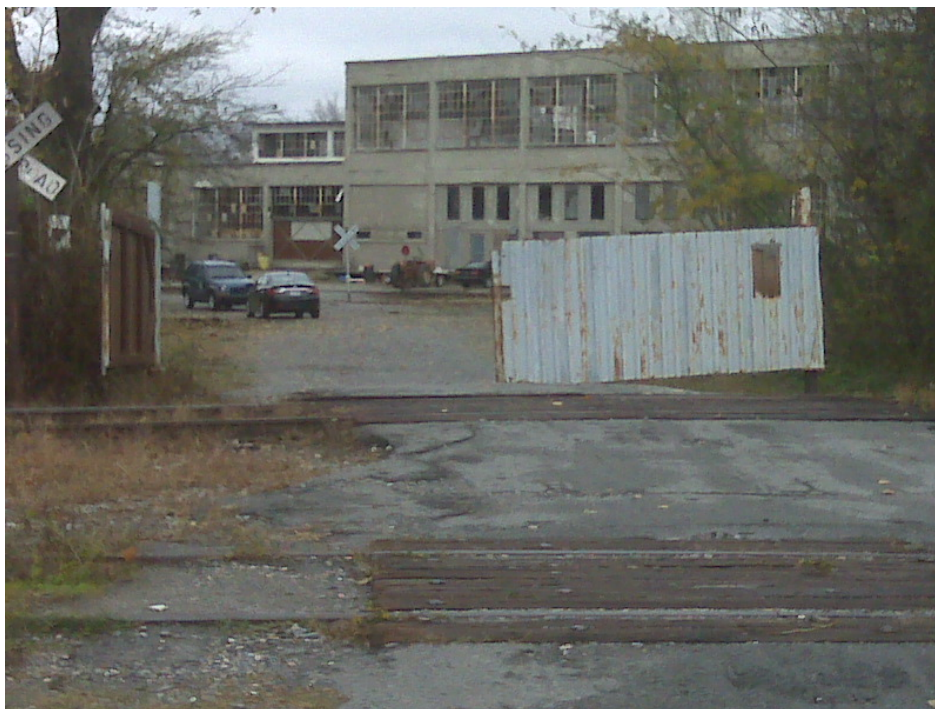
View of entrance to the Former W. R. Grace Facility, past two sets of rail road tracks. Gate can be closed and locked to prevent automobile access.
