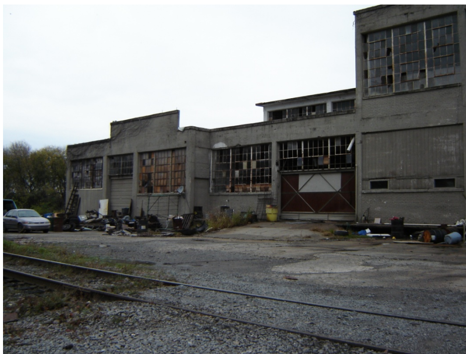
West side of the former loading dock and warehouse at the Former W.R. Grace Facility.
